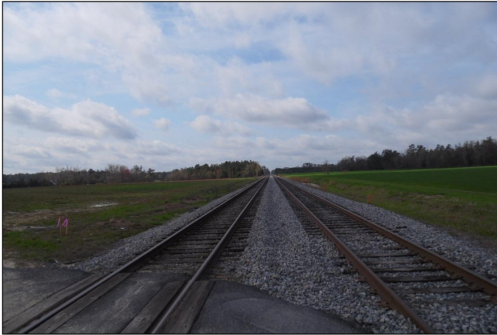
Figure 5. Photograph of the railroad bisecting the Project Area, facing southwest.
